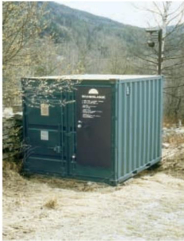
Image 12. Mini fire-station, including water supply in Norway (Source: Norwegian Institute for Cultural Heritage Research)
